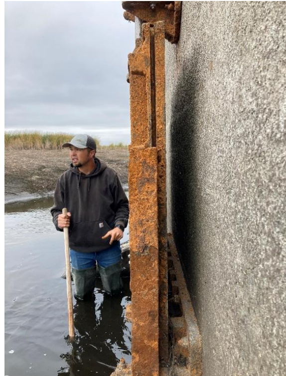
Figure 14 – North Guide Side
