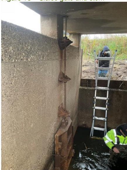
Figure 13 – Sluice gate and stem
