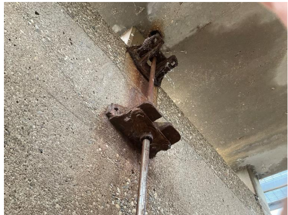
Figure 10 – Sluice gate stem and brackets
