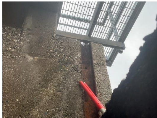
Figure 16 – Stop log channels
