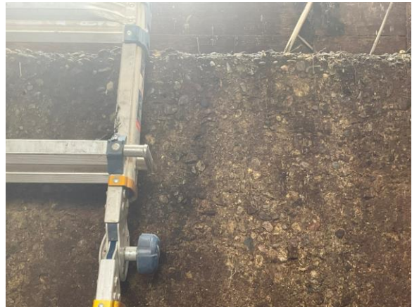
Figure 22 – Crack at outlet with scaling
