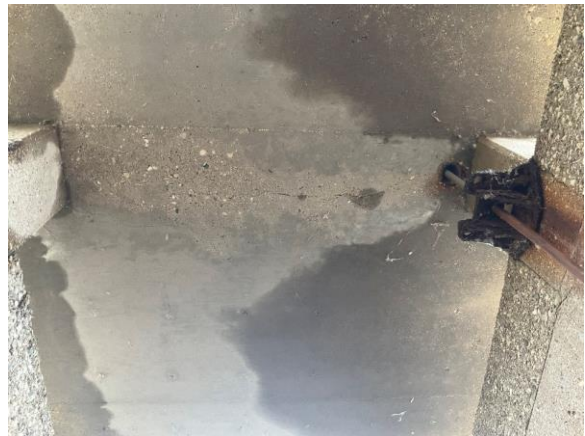
Figure 10 – Sluice gate stem and brackets
