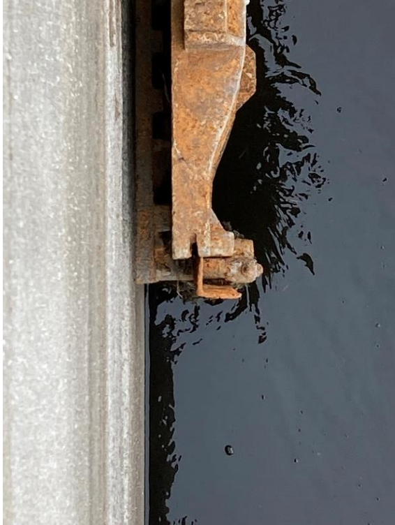
Figure 7 – South Guide Overhead
