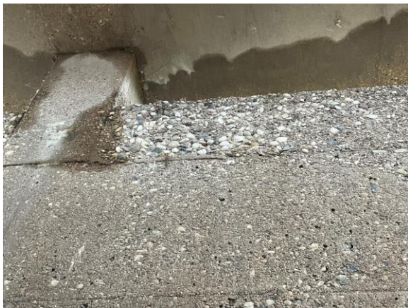
Figure 19 – Concrete scaling
