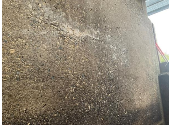
Figure 21 – Concrete scaling
