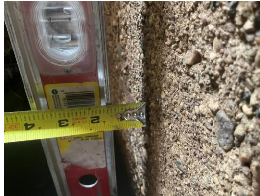
Figure 15 – Stop log channels
