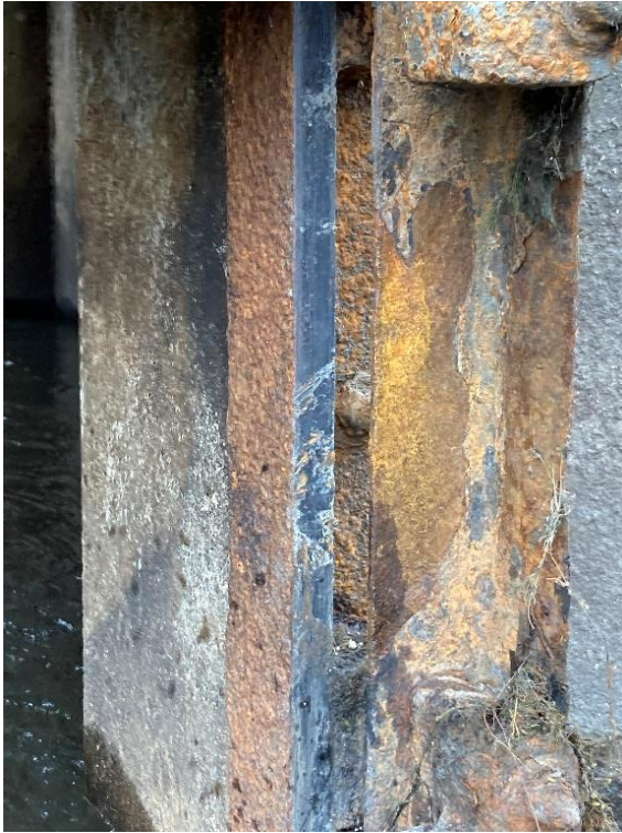
Figure 111 – North Guide Bottom
