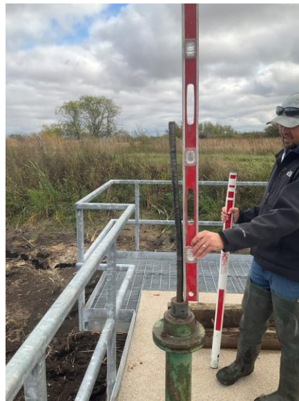
Figure 28 – Upper shaft out of alignment
