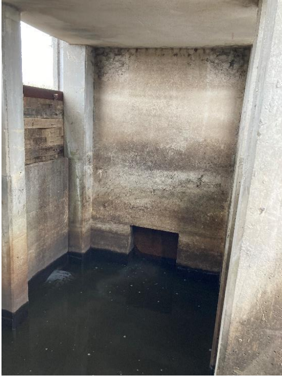
Figure 15 – Sluice Gate Inside Structure
