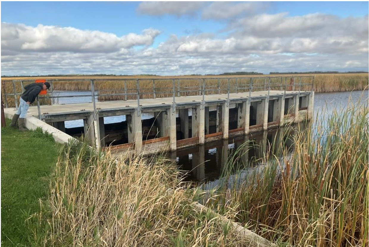
Figure 17 – Outlet Structure South Bays
