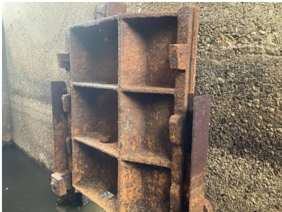
Figure 7 – Sluice Gate
