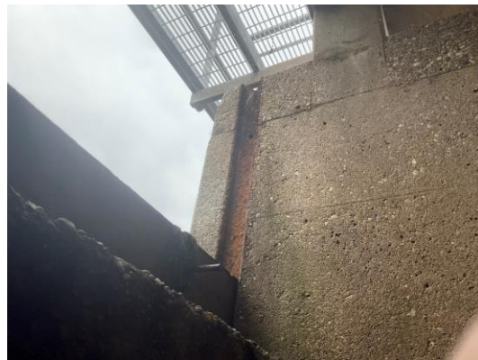
Figure 16 – Stop log channels
