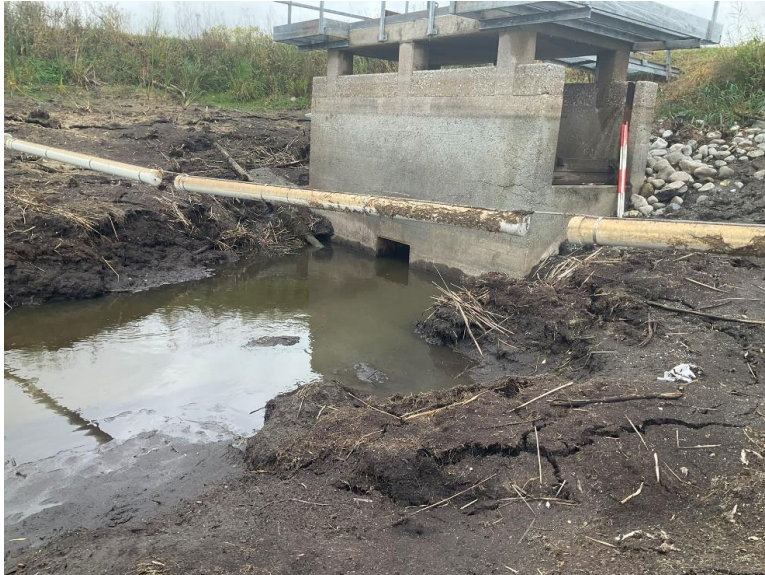
Figure 4 – North side of structure
