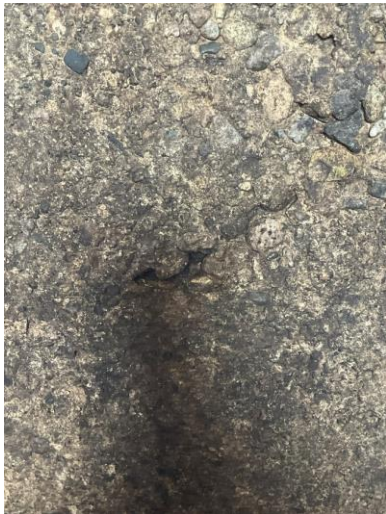
Figure 25 – Upper concrete scaling
