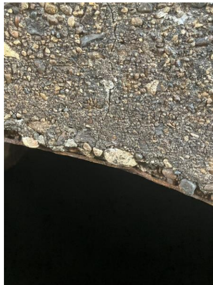
Figure 22 – Crack at outlet with scaling
