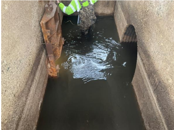
Figure 6 – Sluice Gate
