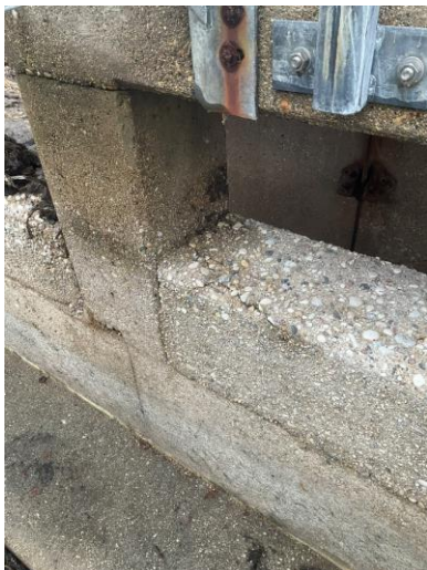
Figure 25 – Upper concrete scaling
