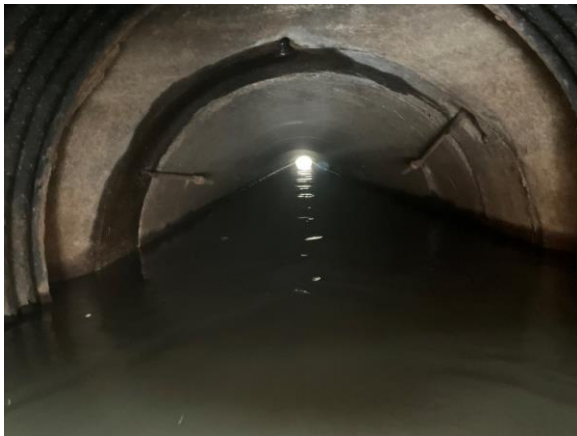
Figure 18 – 48" Outlet RCP Culvert
