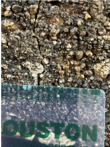
Figure 24 – Concrete scaling
